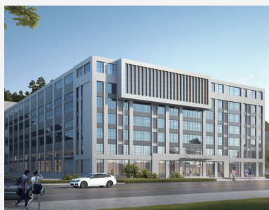
Company Headquarters (Under Construction)
