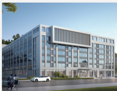
Company Headquarters (Under Construction)
