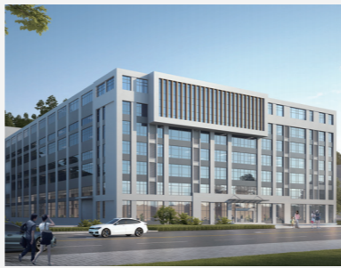
Company Headquarters (Under Construction)
