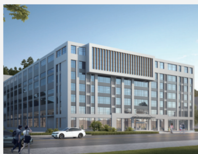
Company Headquarters (Under Construction)
