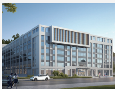
Company Headquarters (Under Construction)
